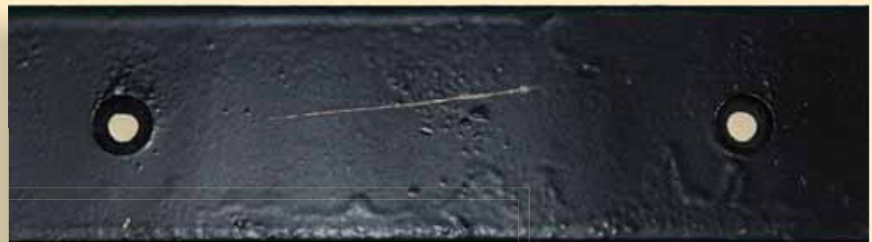
Close up of Deliberate Scratch shows little rust, no rust migration, and no detachment of the surface coating
