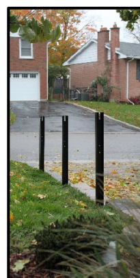
Posts installed Top Notches aligned
