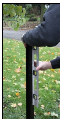
Height & Alignment Check
